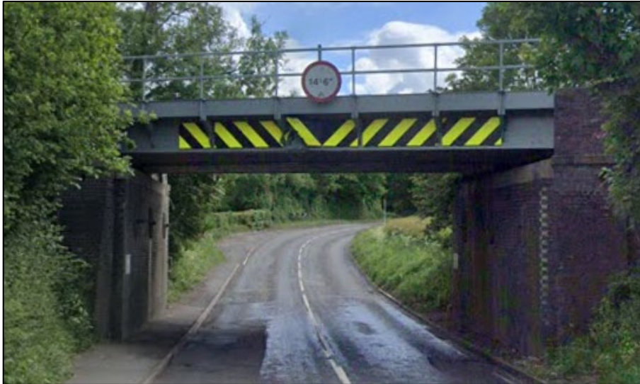
Figure B A5118 railway bridge, view to the east
